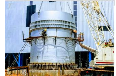
Calciner Hot Stack Erection
